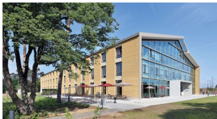
Façade of rammed loam, Alnatura Campus Darmstadt, haas-cookzemmrich STUDIO2050/Lehm Ton Erde Baukunst GmbH
