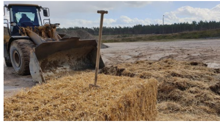
Mixing cob mass, in this case using a wheel loader in a gravel pit in Prignitz district. Photo Dieter Günnewig
