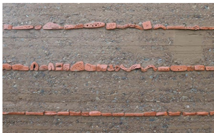
‘Bee stones’ lines integrated into the surface of a wall of rammed loam. Photo Ute Reeh
