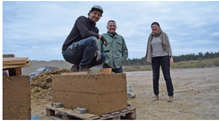
Cob block after removal of the reusable formwork. Photo Fabian Lehmann
